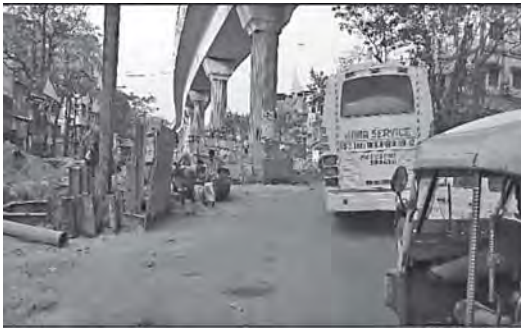
Plate 3: Road diversion at Silpara
