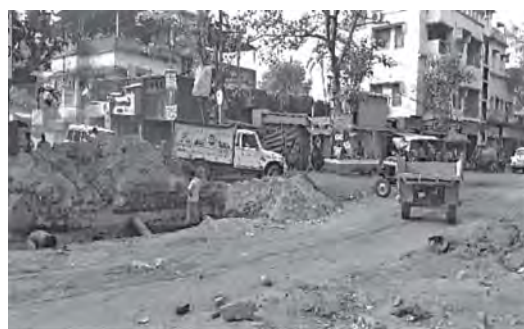
Plate 4: Excavation at DH Road for Metro construction
