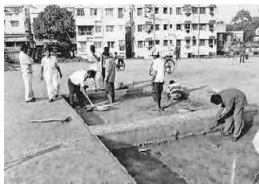
Fig. 5. Excavation is in the progress of the Dumdum mound. ASI, Kolkata, 2001.
