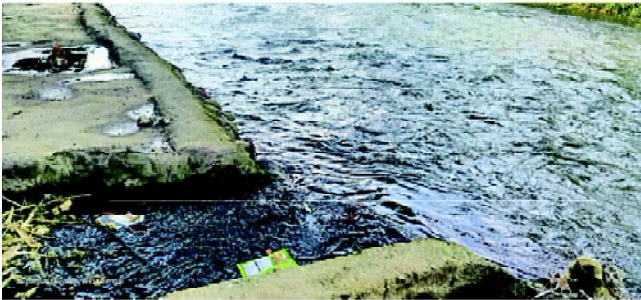
Photo 16: Domestic drain outlets are discharging at Chamta
