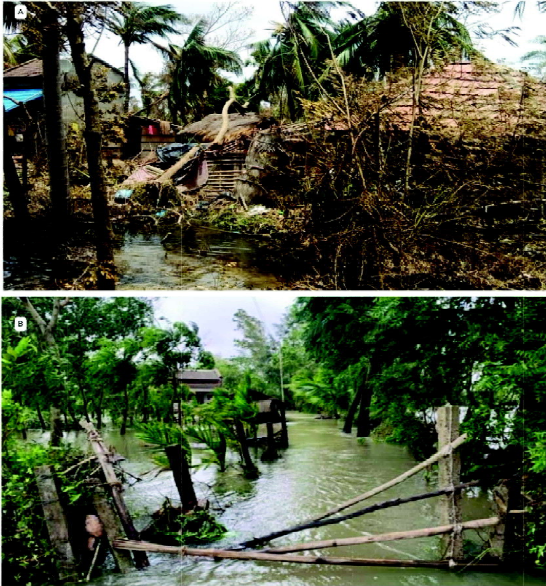
Photo plate-1: Effect of Amphan & Yaas (a) Houses damaged during post Amphan Cyclone in Patharpratima, South 24 Parganas (b) Houses damaged during the post Yaas Cyclone in Gosaba, South 24 Pargana.
