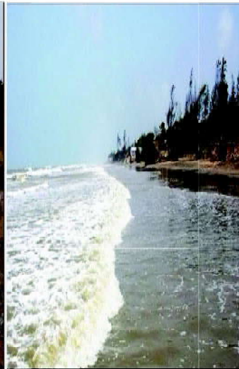
Fig.12 Coastal erosion due to cyclonic storm at Digha
