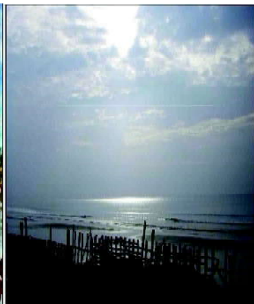
Fig.15. Sankarpur beach protection groins to prevent erosion
